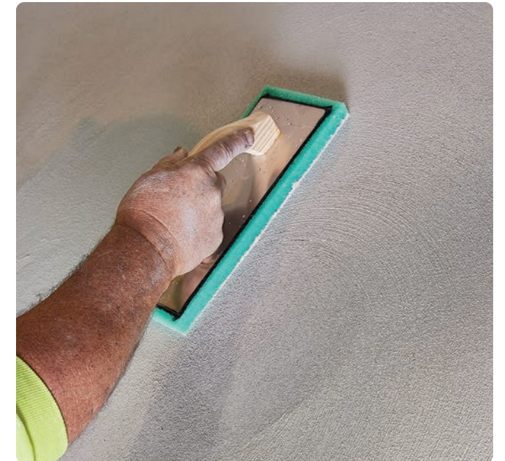
Finish (second) coat (Smooth or Texture Finish)
