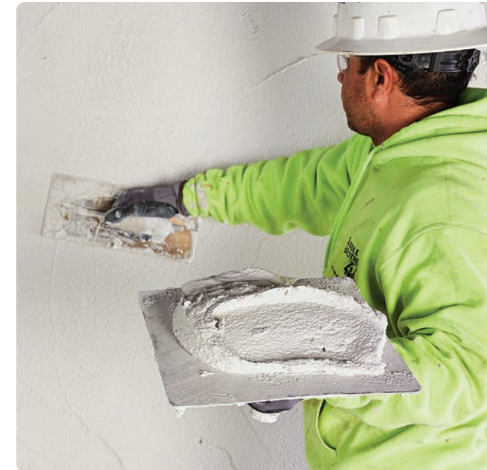
Base (first) coat on Kal Kore Plaster Base
